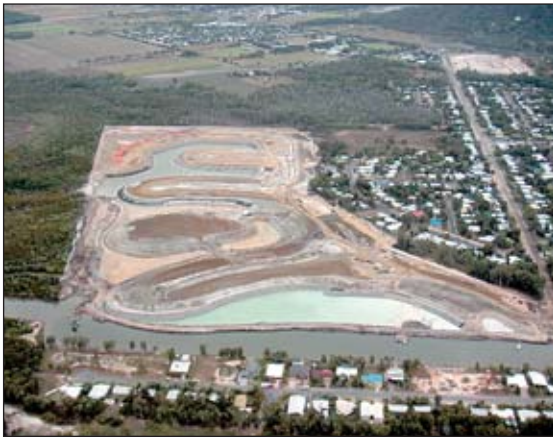
Aerial view of Bluewater during construction.
